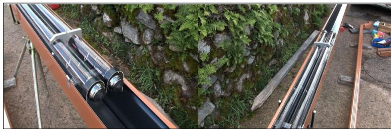
Figure 5. H2OSS® Concept with Narva vacuum solar integration into the building's gutters
