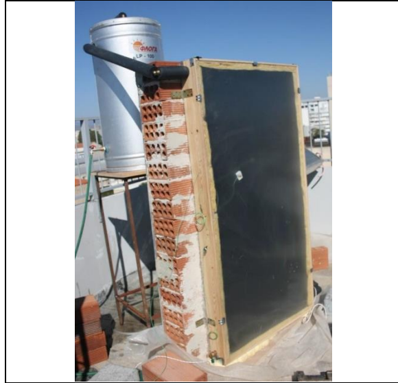
Figure 2. Prototype construction of the integrated hot water collector
