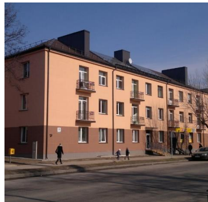
Fig. 5. Residential building after retrofitting
