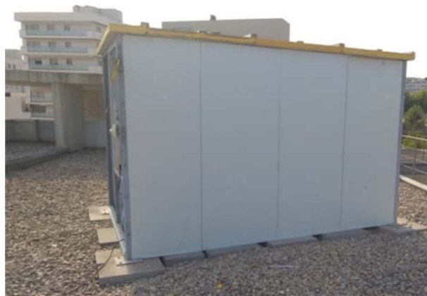
Fig. 1. The outdoor testing unit (University of Lleida, Spain).
