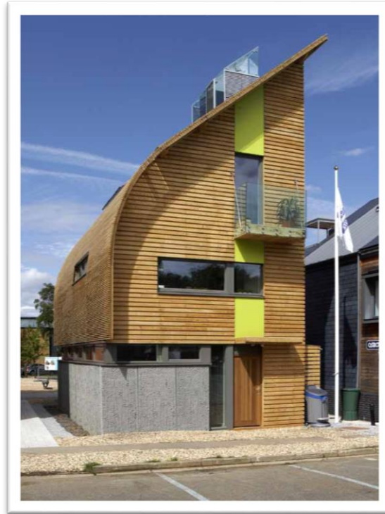
BRE zero carbon house UK includes photovoltaics, biomass boiler and 'wind catcher'
