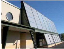
District heating, Sweden
