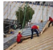
Significant back panel insulation, Portugal
