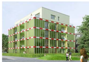
Integrated photo-bioreactor, Germany
