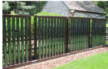
All-ceramic solar collector, China
