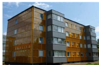
Solar-comb insulation, Austria
