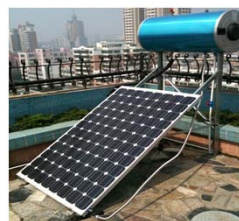
TEΣ PV/T SOLAR WATER HEATING SYSTEM
